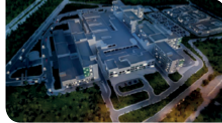
Eskişehir Şehir Hastanesi, Eskişehir Eskişehir City Hospital, Eskişehir
